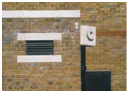
When unavoidably interior to the walls, JOA gutters are always fitted with prominent overflow outlets. This was a rainwater hopper, and overflow, in ballidon limestone concrete, to the transformer building.
