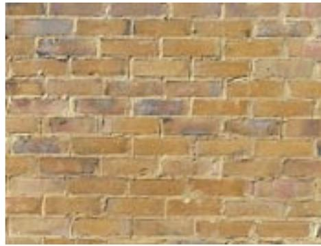
At Poyle the excess mortar 'fat' was cut off, flush to the bricks, with a single upward strike of the trowel. The joints were not 'struck' that is pushed in to solidify their surface as such a protection of the joint betrays an ignorance of how stock bricks suck rainwater OUT of joints.
