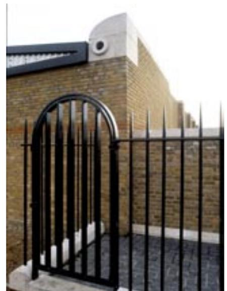
The iconography of a London house-railing needs no great erudition to decipher. They are rows of black iron spears bedded into stone walls with molten lead. JOA used the same notion, for a gate and fence to the canal, only with blade-type points to stay within the law.
