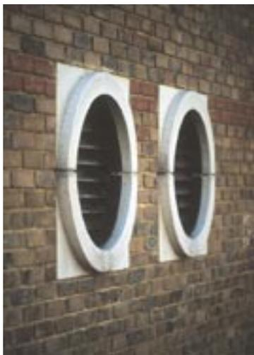
Ventilation extracts. Nothing was allowed to penetrate the masonry skin unless it was fortified by a massive and solid cast ballidon limestone grommet.
